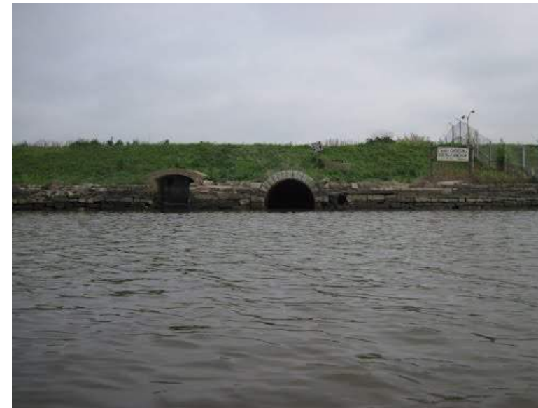
example of outfall at Anacostia River
