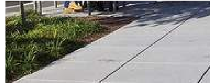
concrete sidewalk - Half Street. & T Street
