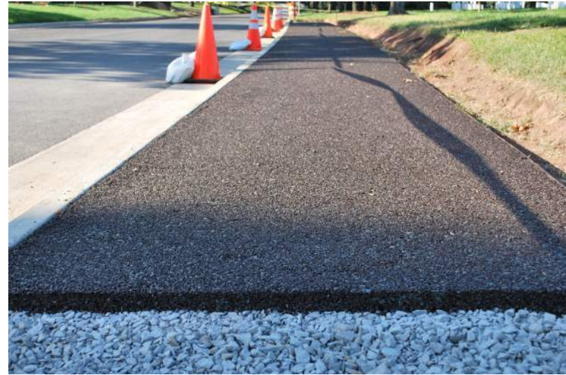
river walk trail over critical roots zones - flexi-pave
